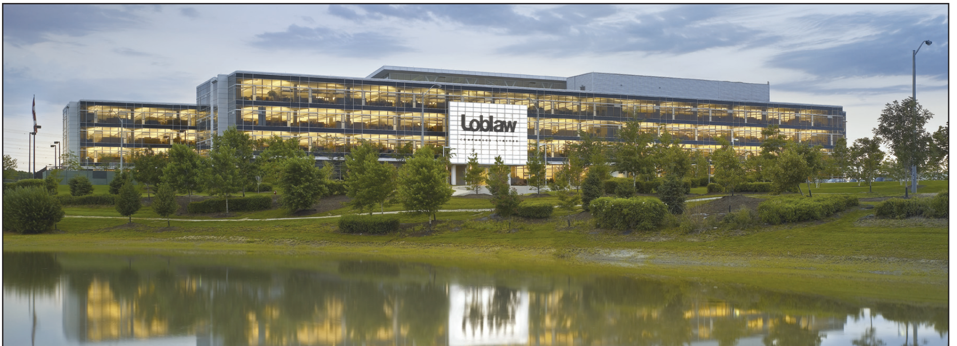
The Loblaw Companies Limited HQ building is arranged in two parallel, four story wings, offset from one another and oriented with their long sides facing due south to take maximum advantage of solar exposure.
