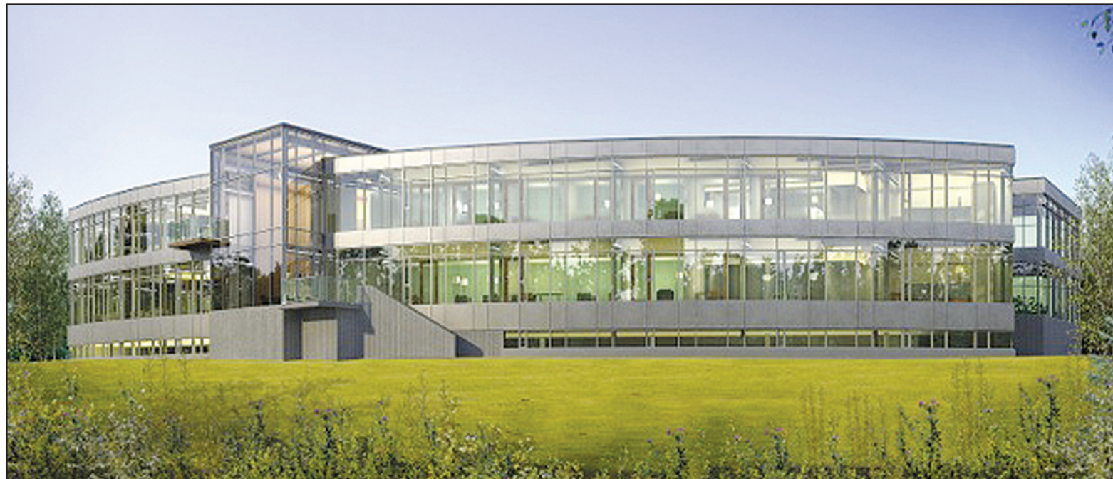
The Fishkill LandWorks Professional Center is preparing for an end of year groundbreaking and is seeking LEED Platinum certification.
